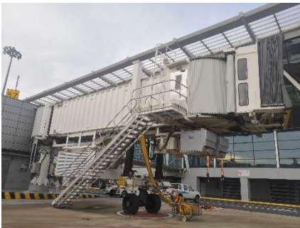
PBB/Ground Mounted Cable Reel 2x90KVA
